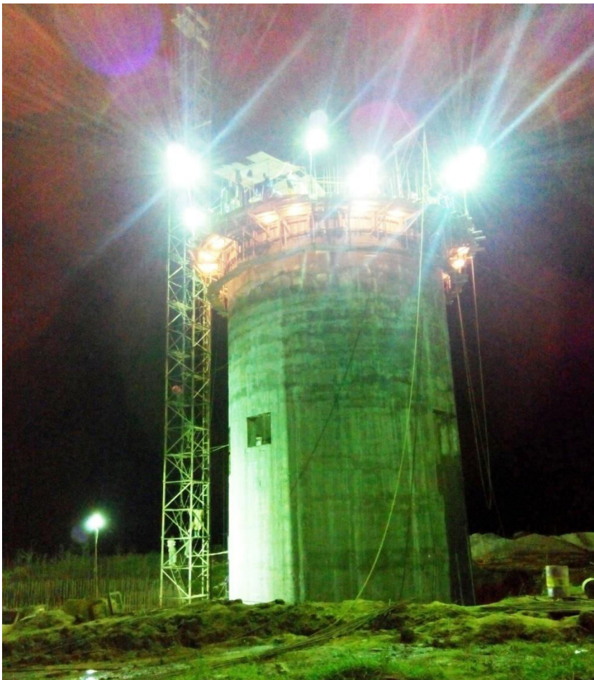
OPC Silo under construction at Maweni Limestone Ltd., Tanga, Tanzania
