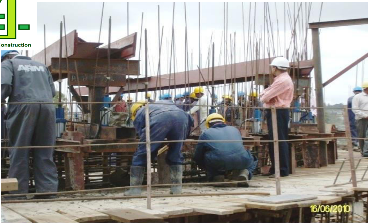
Clinker Silo construction work in progress at ARM Cement, Nairobi, Kenya
