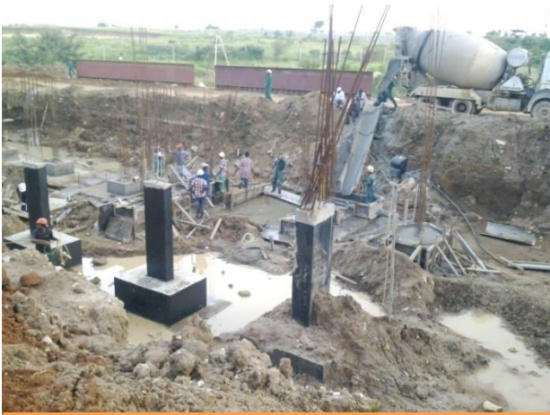
CCR Building footing under construction at Maweni Limestone Ltd., Tanga, Tanzania
