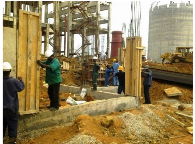
CCR Building under construction at Maweni Limestone Ltd., Tanga, Tanzania
