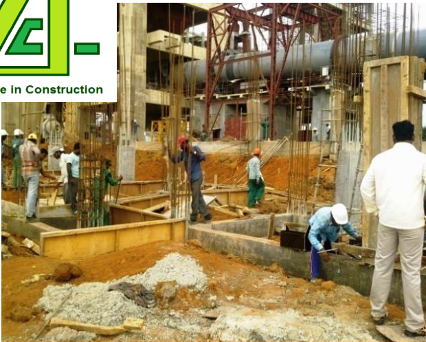
CCR Building construction at Maweni Limestone Ltd., Tanga, Tanzania
